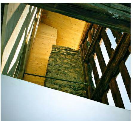
IN OUESTA PAGINA, IN ALTO, SI NOTA COME IL RIVESTIMENTO IN LEGNO DELLA VECCHIA STALLA SIA STATO PRIVATO DI OGNI SECONDA TAVOLA PER DARE PIÙ LUCE AL CORRIDOIO. IN BASSO, SI PUO' RICONOSCERE UN PILASTRO PORTANTE DELLA STALLA. ON THIS PAGE, ABOVE, EVERY SECOND FIR PLANK HAS BEEN REMOVED TO GIVE MORE LIGHT TO THE PASSAGE. BELOW, IT'S POSSIBLE TO SEE A PILLAR OF THE STABLE.
